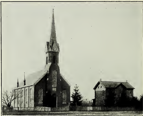
ST. MAURICE'S CATHOLIC CHURCH.
